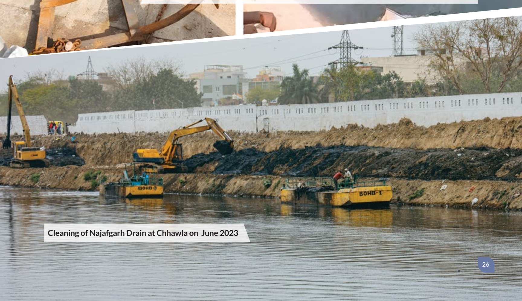
A unique Partial Gravitational De-silting process started in Najafgarh Drain in August 2022
