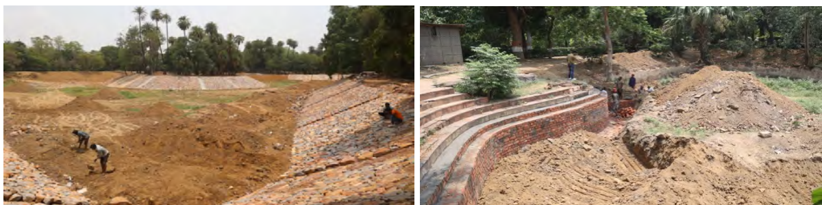
Image : Restoration work underway at Roshanara Bagh Lake
