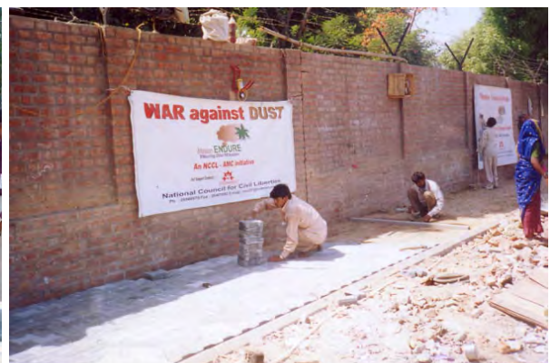
Work in progress at 132' ring road, Vastrapur
