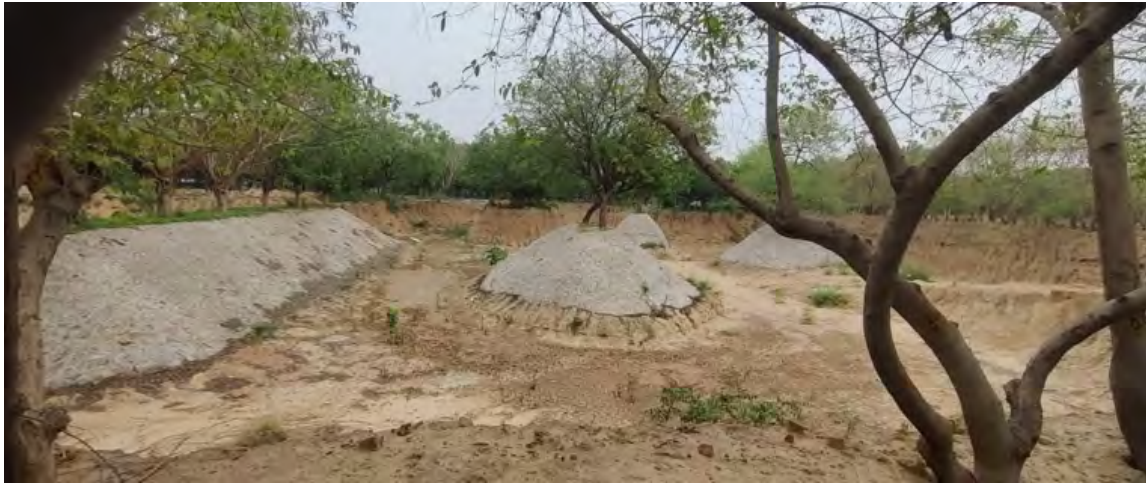
Image : Rejuvenation of a water body underway at Sector – 20, Dwarka
