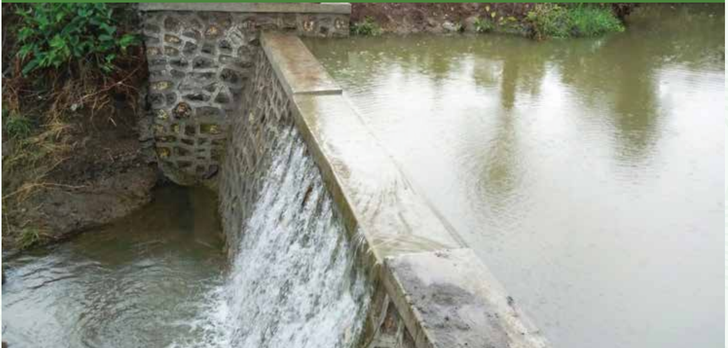
A check dam constructed at KVIC's Nagpur centre
